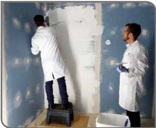
Application of Dulux Trade Plus ThermoCoat+
